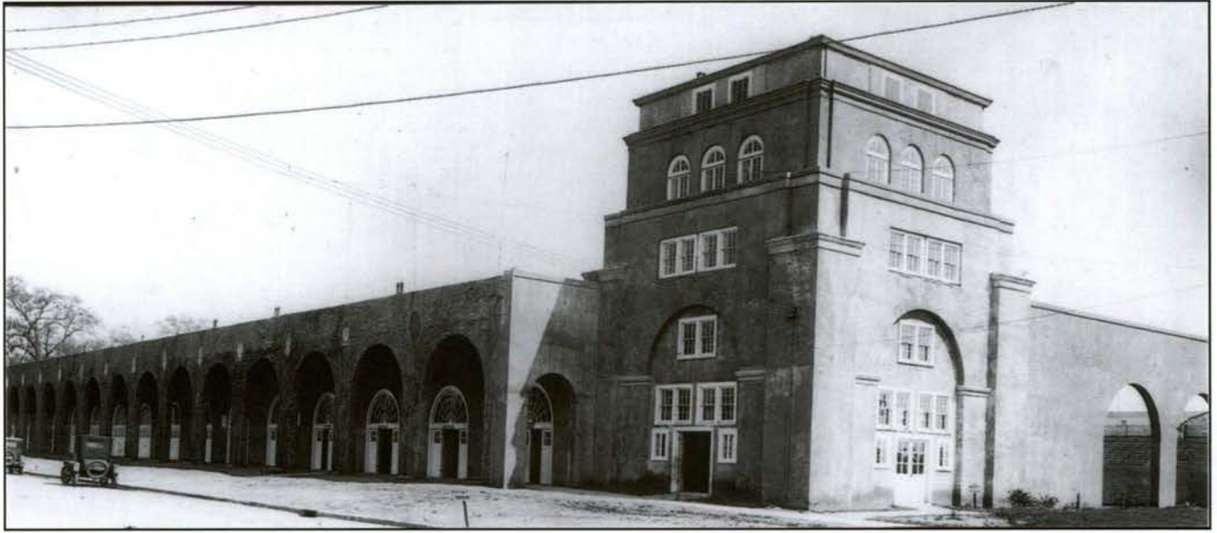
Figure 111: Doughboy Stadium is built of reinforced concrete in the Spanish Mission style. Construction costs were paid by soldiers in tribute to fallen comrades from World War I.
